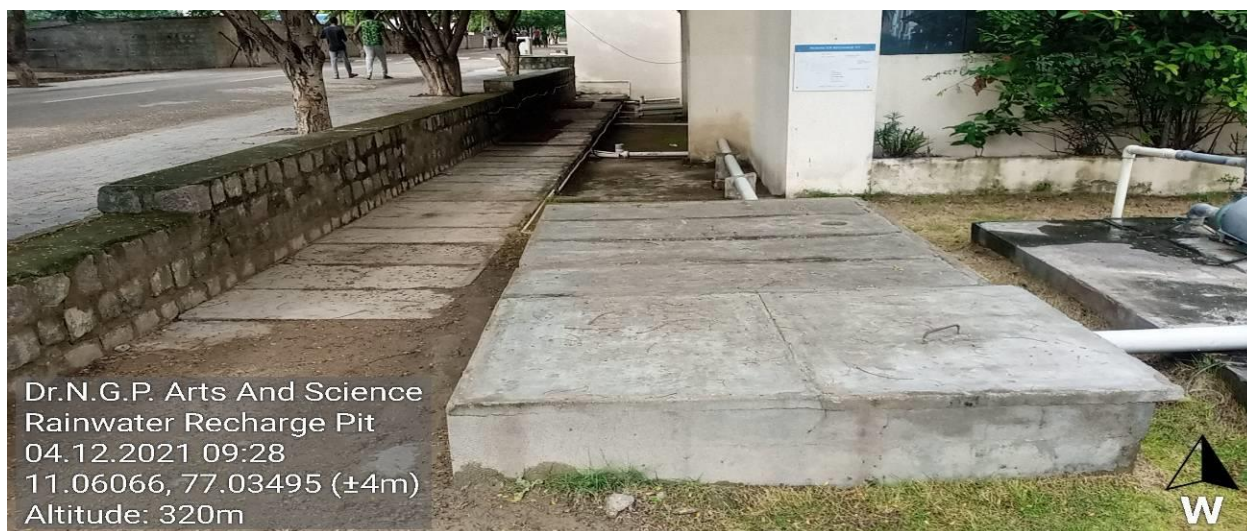
Rainwater recharge pit at B1 Block Front Side
